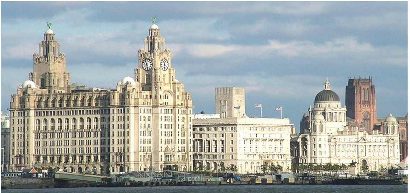
Liverpool Pier Head, with the Royal Liver Building, Cunard Building and Port of Liverpool Building
